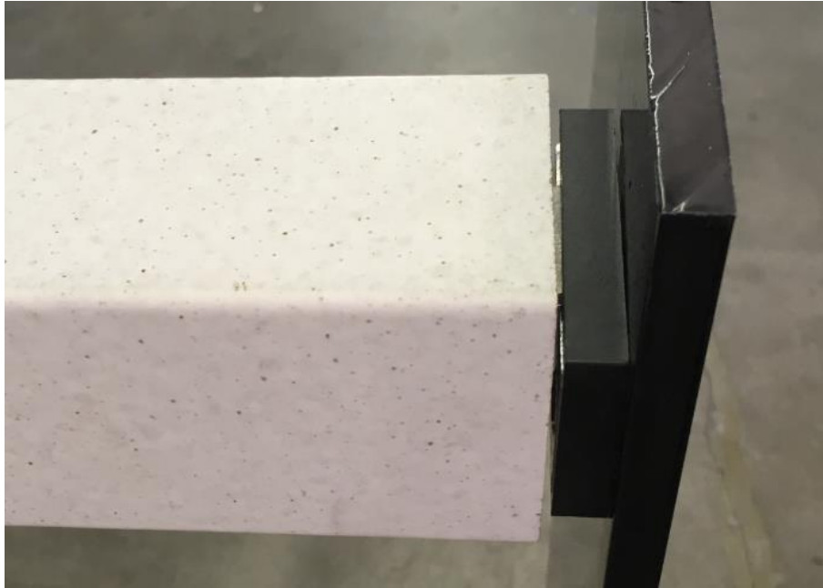
Figure 11: assembly with securing clip installed
