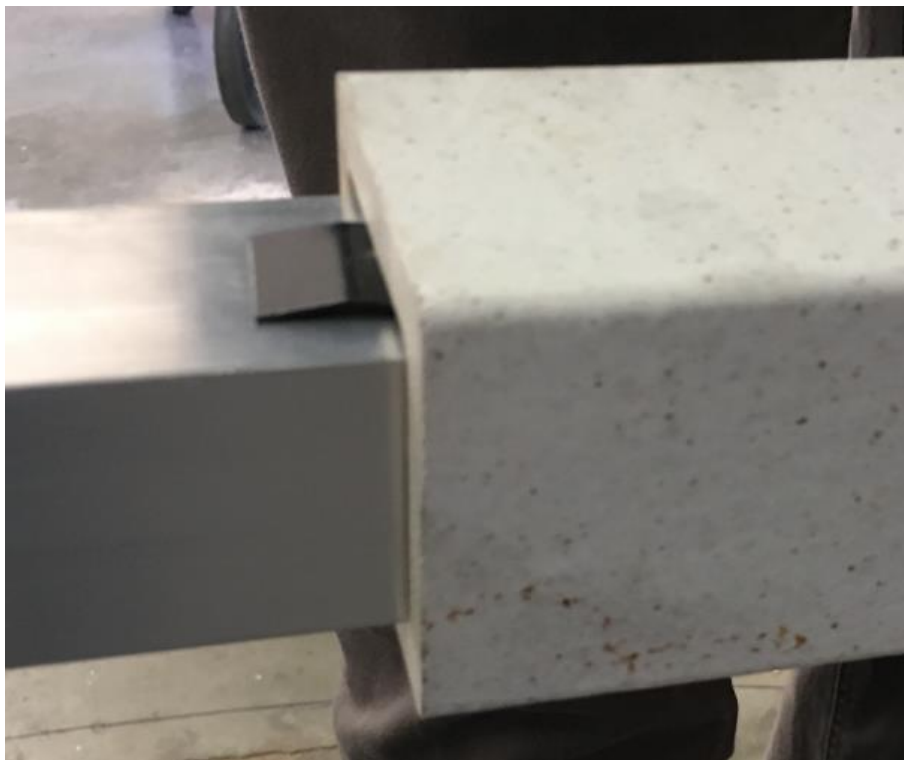
Figure 7: spring clip during installation
