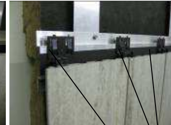
put the panels into the preassembled clamps. at the edging use the edge-clamp Art. Nr. 684 ... for further fixings use the twin-clamps Art. Nr. 680
