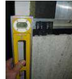
put the panels into the preassembled clamps. at the edging use the edge-clamp Art. Nr. 684 ... for further fixings use the twin-clamps Art. Nr. 680
