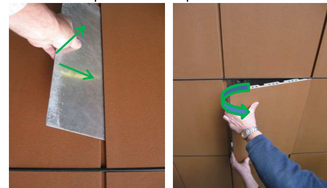
replacement of a panel
