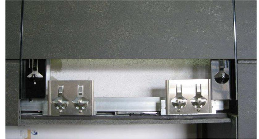
At a panel length above >600mm 2 couple of hooks have to be installed right and left next to the vert. T-profiles.
