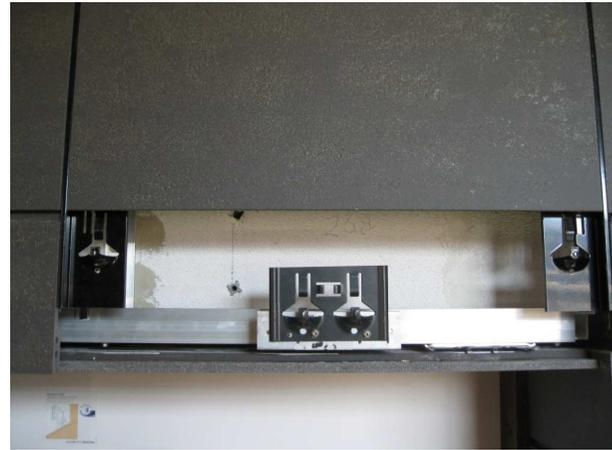
Install a couple of hooks onto a special prepared substructure in the centre of the panel. Max. panel length 600mm
