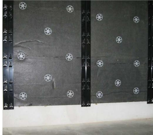
distance bottom line panel to top of the hook = 63mm
