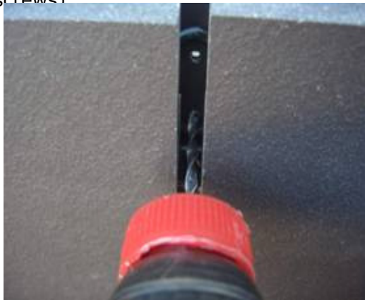
drill the holes in the joint ... (screws)
