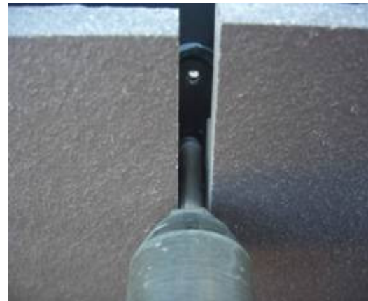
... and fix it with rivets(or
