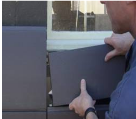
slide panel in the lips of the clamp
