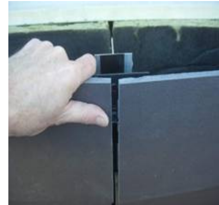
install always a couple of panels
